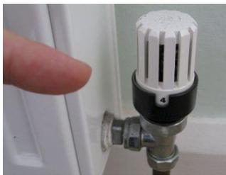
**TRV'S:** In some properties TRV'S are fitted on one side of the radiator (see the photograph to the left) \*please note, these are not in all of our properties. Thermostatic Radiator Valves enable you to control the heat of individual radiators in your property. If you're too hot in your room for instance you can decrease the temperature of your own radiator, while leaving the one in the bathroom on a higher setting if it's colder in there.
